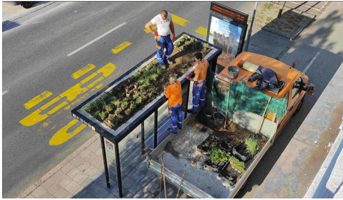
Installation of green roof on bus stop
